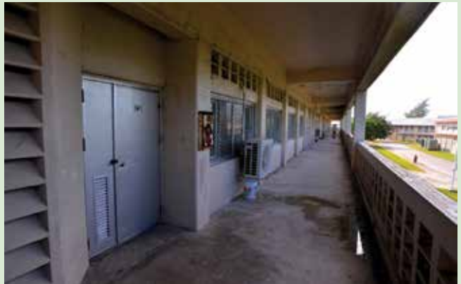
Figure 3-12. All exterior doors leading to the shelter areas should be sturdy metal or solid wood doors, with quality hinges and door latches to secure the shelter during high winds with potential debris impacts
