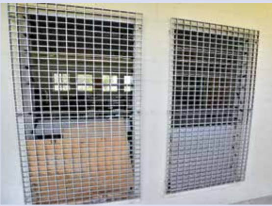
Figure 4-35. Another option for window protection is this aluminum security screen seen on a few schools such as Marshall Islands Middle School. The screen allows in light, and the openings are sufficiently small to stop most debris. The framing is bolted into the concrete masonry unit wall. While stronger than the screen in Figure 4-34, it is also more expensive. This is good window protection for houses with CMU walls (see Figure 4-1).
