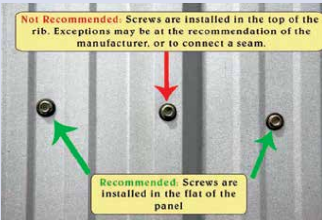
Figure 4-24. Some roofs in Majuro have flat sections that differ from undulating roof sheets shown in Figures 4-20 and 4-23. In this case, fasteners to the purlins should be in the flat lower flat portion of the panel. Photo courtesy of Christian Oakes, IOM.
