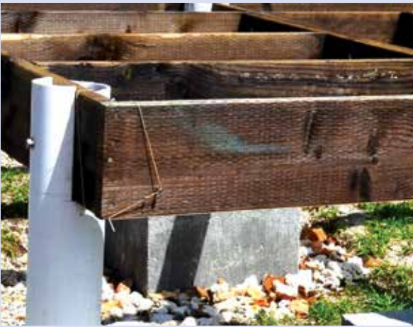
Figure 4-36. Example of ACZA wood suitable for use in the marine environment. Note the cuts or incisions on the surface to increase penetration of the chemical treatment. Because the chemicals in this wood are very corrosive, as well as the marine environment itself, stainless steel fasteners are used to attach the column to the wood joists (support for the flooring). Photo courtesy of Ben Chutarro.
