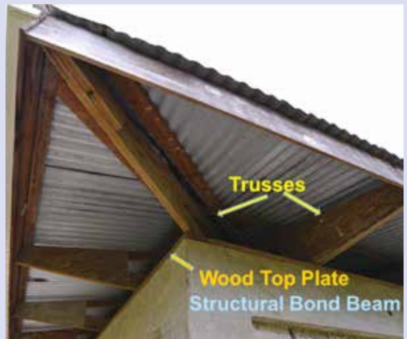
Figure 4-3. On top of the concrete structural bond beam is commonly a wood top plate, consisting of 2 inch by 4 inch lumber. On top of the wood plate are the trusses. To prevent wind damage during a storm, there must be a strong connection from: (a) the wood top plate to the structural bond beam; (b) the trusses to the wood top plate; (c) purlins to the trusses; and (d) metal corrugated roof to the purlins.
