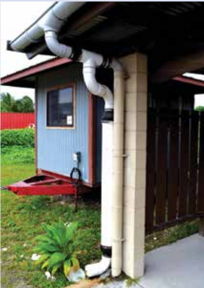
Figure 4-54. First-flush systems can be ordered or they are easy to create yourself. Ask your local hardware store if you have any questions about materials or how to build one. The systems are sized for the size of the roof. As a general rule, and from existing literature, the diversion pipe must catch 5-10 gallons of water per 1,000 square feet of roof area (see University of Hawai‘i Mānoa pamphlet and website). See Table 4-5 to see the relationship between first flush diverter pipe diameter width, length and amount of water to collect.
