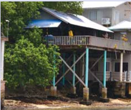
Figure 4-40. This house in Majuro was elevated to prevent damage from wave inundation and flooding. This is an extreme example of elevation of structures. Many houses in Majuro have been elevated a more modest amount (see Figure 4-41). This house has a spread concrete footing (see Figure 4-42). The brown wood members forming the X pattern are cross bracing to provide additional lateral support of the structure.
