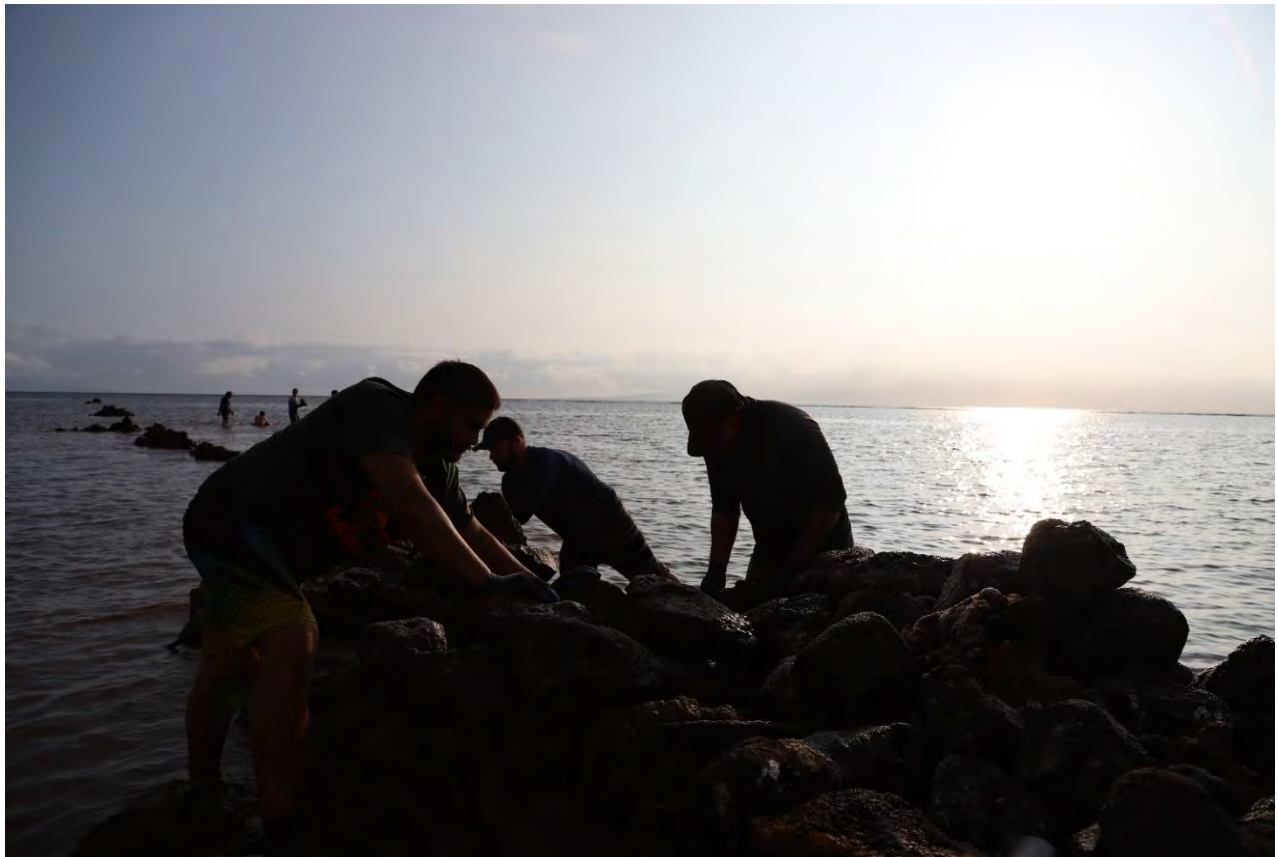
Building wall at Wai'ōpae. Photo credit: Kanda.
