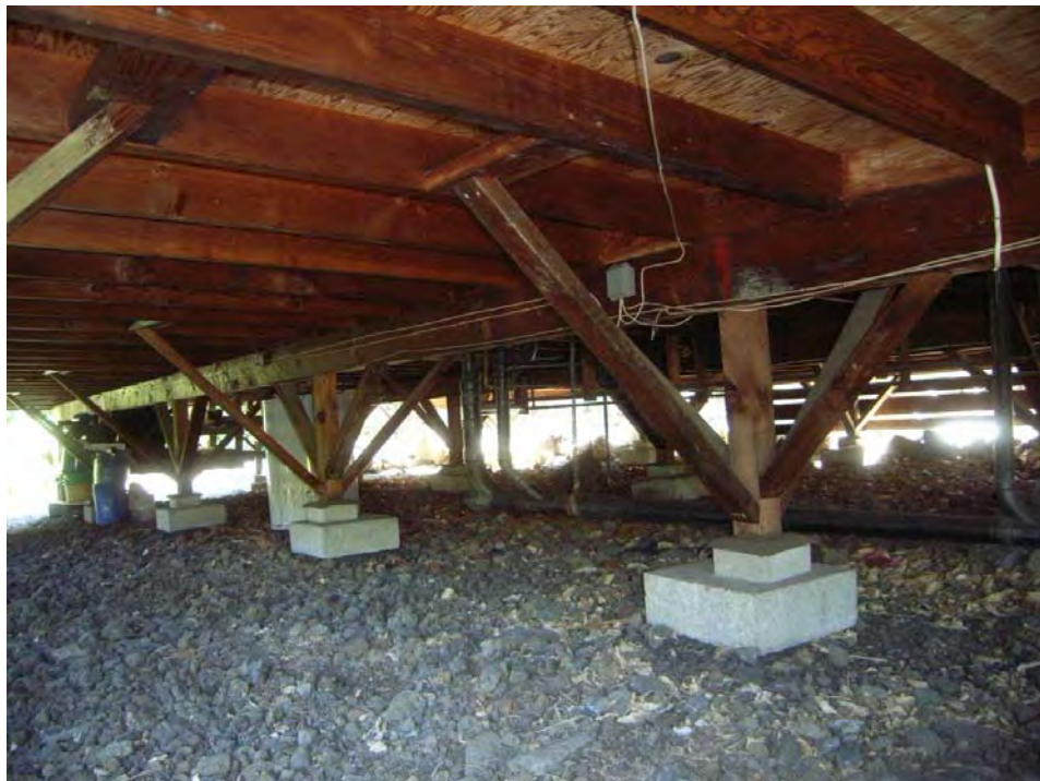
Figure 2-1. Typical post and pier foundation
