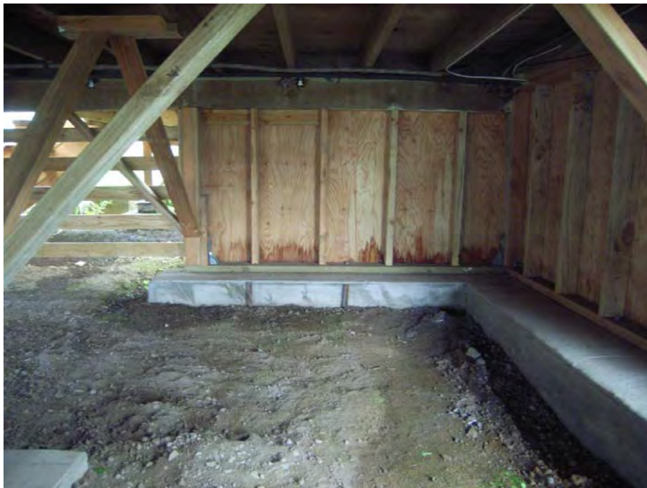
Figure 6-1. Typical corner plywood shear wall providing lateral strength and stiffness to a house with a post and pier foundation system
