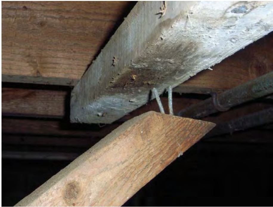
Figure 2-7. Nail pullout failure of a post brace
