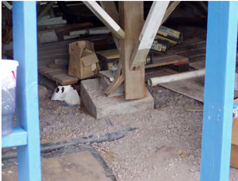
Figure 2-5. Lack of post anchorage resulting in walking and splitting of post as it unseats from foundation blocks
