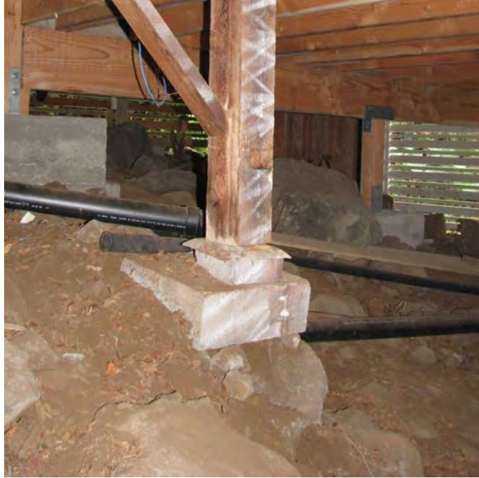
Figure 2-3. Undermined pier due to unstable soil conditions
