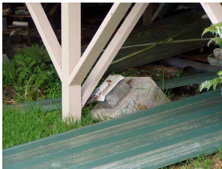
Figure 2-4. Lack of post anchorage resulting in sliding of post and toppling of foundation blocks
