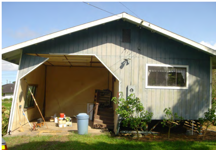
Figure 2-6. Lack of post anchorage resulting in unseating and lateral displacement of posts
